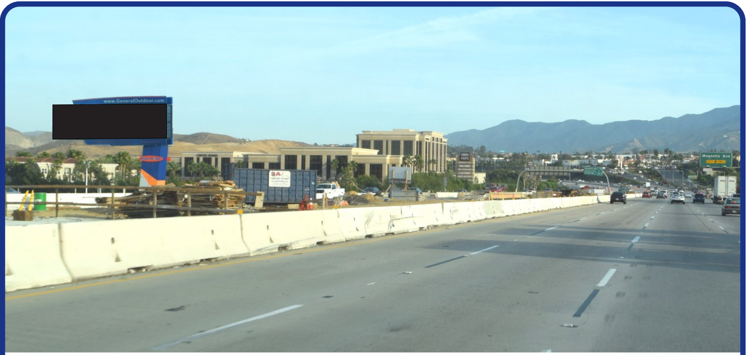
I-15 & 91 Fwy Interchange
